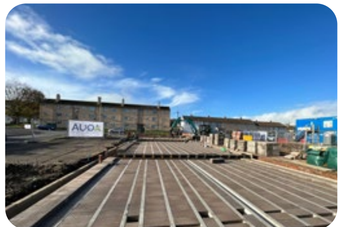
Work has started to transform the former pub site
